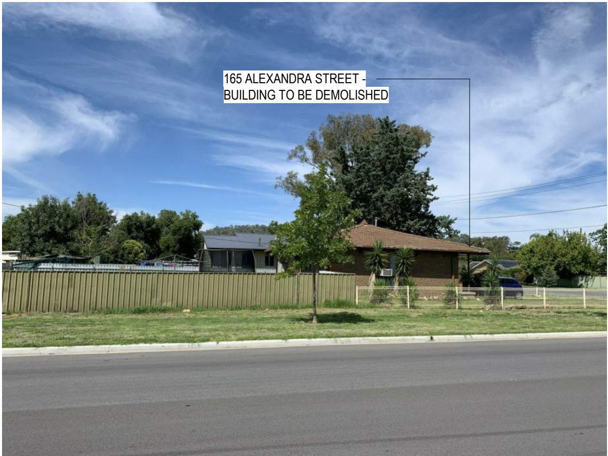
165 ALEXANDRA STREET ELEVATION VIEW
