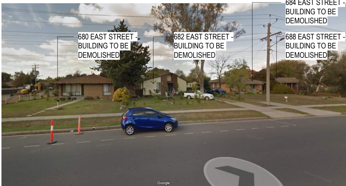
680 - 688 EAST STREET ELEVATION VIEW
